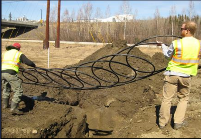
Installation of Slinky Loop
