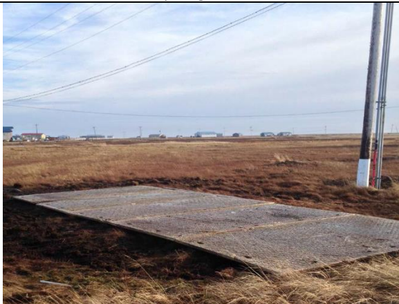
Site mats positioned awaiting the battery
