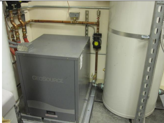
Installed 3 ton heat pump
