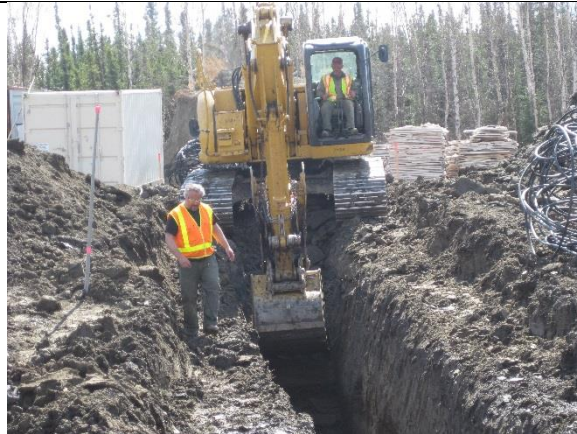
Digging the trench for the coil
