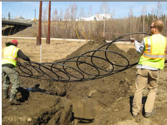
Installation of the slinky loop
