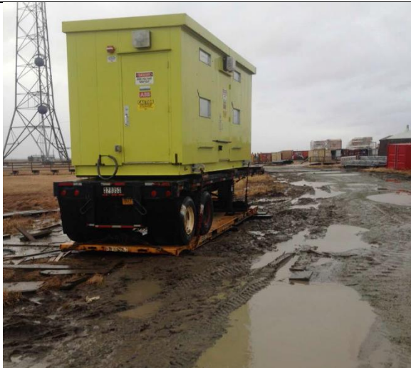
Battery and enclosure awaiting freeze up
