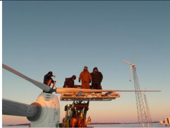
Installing turbine blades
