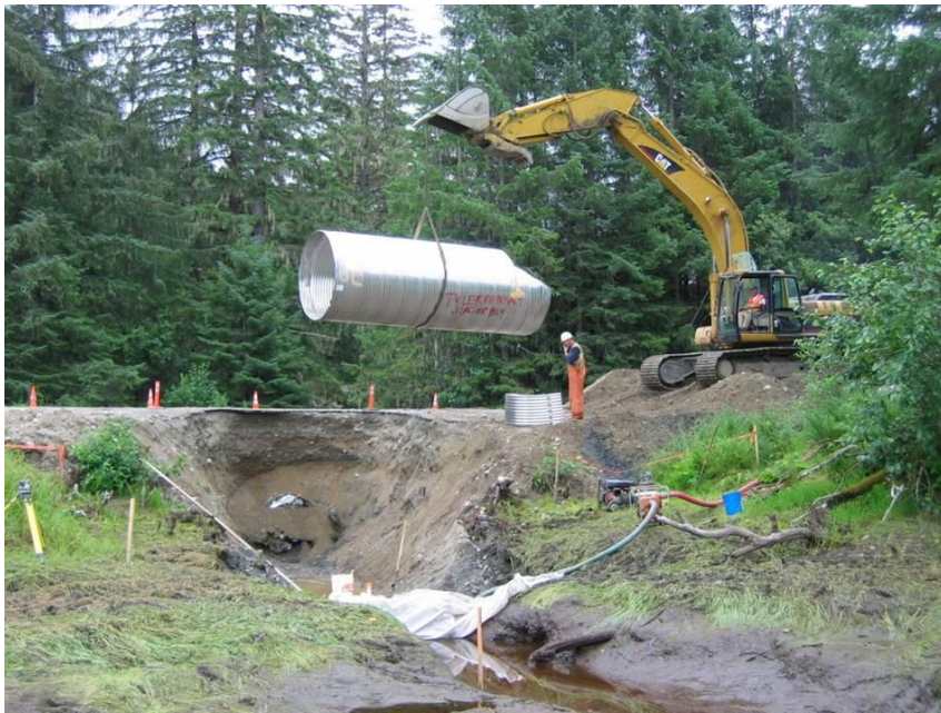
Culvert Installation
