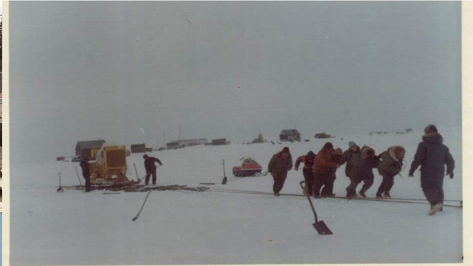
2. An 8000 lb. generating unit is placed upon a sled by block-and-tackle and manpower.
