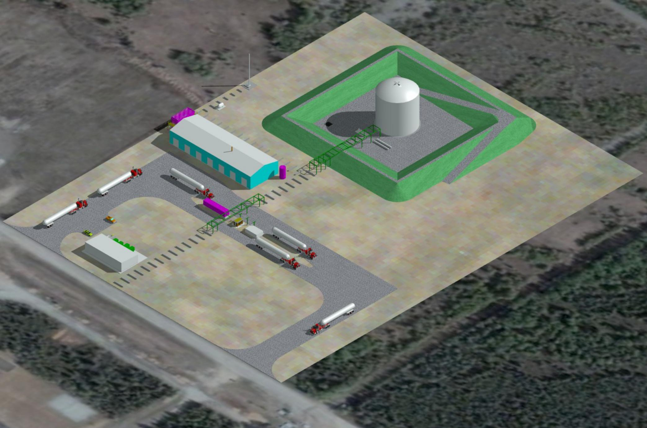
**Facility Description:** LNG truck receiving and offloading, LNG storage, LNG truck fueling, HP & LP vaporization and sendout for separate users (usage) and associated systems -- building, structural supports, piping, electrical, instrumentation & controls adequate for the environmental conditions expected.
